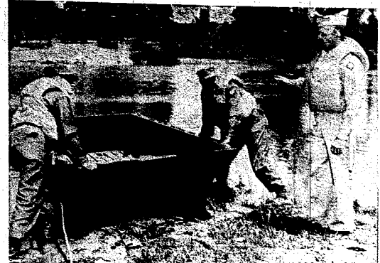
BEGIN BRIDGE . . . Work is begun on a floating bridge by U.S. Army Reserve officers from Albuquerque, N. Mex., members of the 4153rd USAR School. The officers are receiving instruction in the third year company officers course, Engineer Branch. Left to right are Major Severn Starzynski, Capt. John L. McCormick, and Capt. William J. Cooke. Capt. Cooke is a member of the staff of the Albuquerque USAR School and is serving as an instructor during the unit's training.
